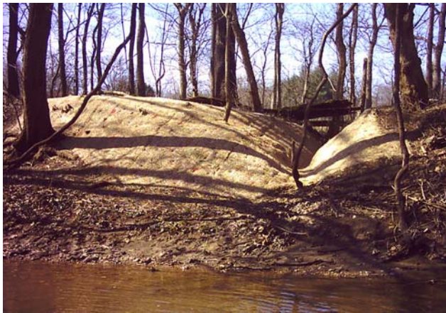
▲ During: Streambank in north woods cleared of bush honeysuckle and wintercreeper. Biodegradable erosion matting was installed to help secure native seed mix. Native bare root whips were later planted into the matting material. (March 2006)
