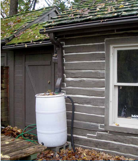
A rain barrel collects rain from the roof of the LREC cabin. Photo by Leslie Memula.
